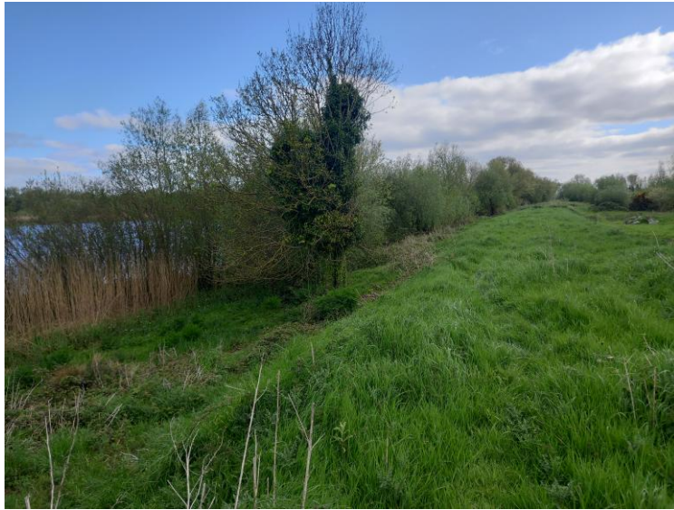
PLATE 13-9 EMBANKMENT TO THE NORTH OF CORCANREE PS ALONG THE SHORE OF THE SHANNON ESTUARY
