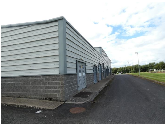
PLATE 13-12 EXISTING BUILDING WITHIN LIMERICK WWTP WITH NEGLIGIBLE SUITABLE ROOST FEATURES FOR BATS
