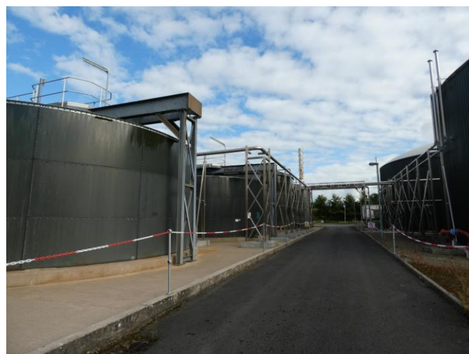
PLATE 13-13 EXISTING WWTP INFRASTRUCTURE WITH NEGLIGIBLE ROOSTING SUITABILITY FOR BATS
