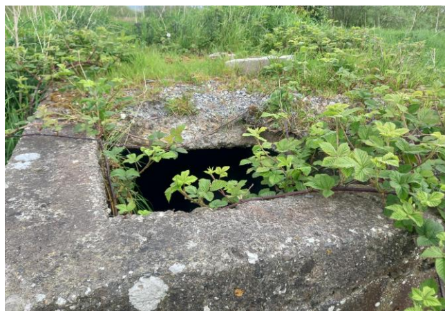
PLATE 13-19 UNDERGROUND CAVITY LOCATED ADJACENT TO THE PROPOSED CONSTRUCTION ACCESS ROUTE FOR THE STORM TANK.
